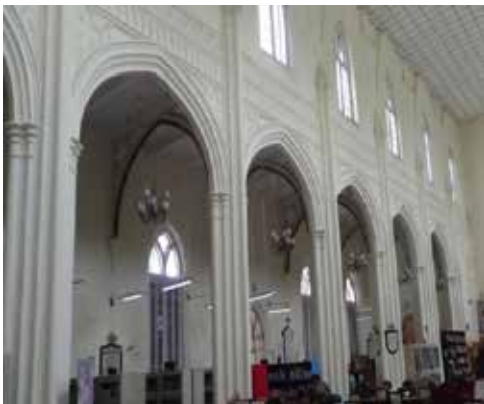
INTERIOR OF CHURCH AFTER RESTORATION
