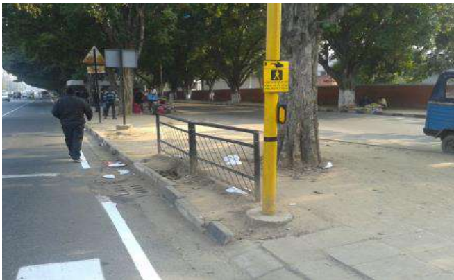
Fig.5. Railing Provided at the Location
