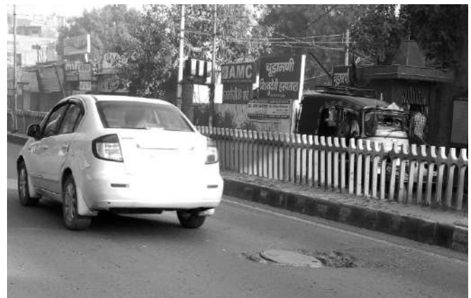
Fig. 4. Sewerage Manhole Coming in the Midway of a City Road
