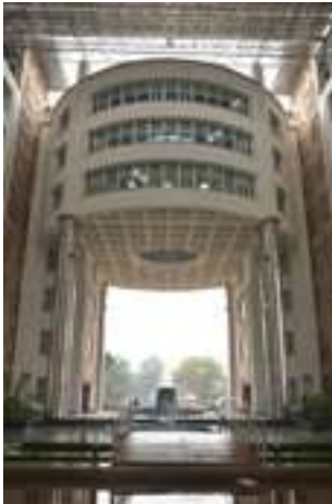
Fig. 3: Covering of Central Courtyard
