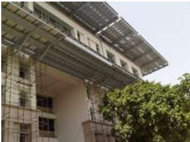
Fig. 4: Extended Roof at 4 th floor and Roof Level
