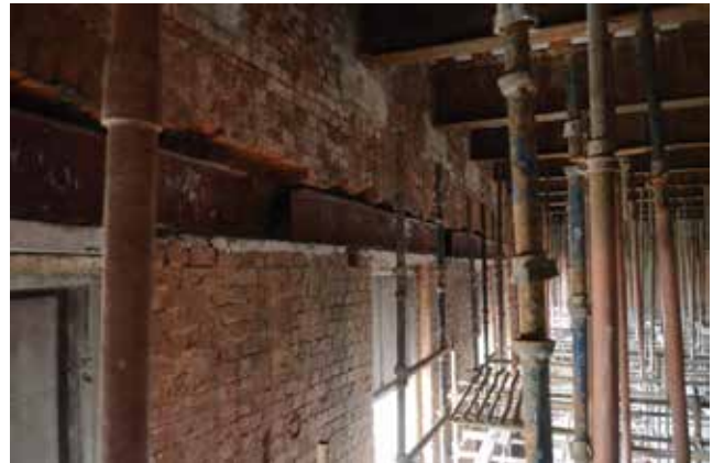
Fig.2: Retrofitting works at Writers Building, Kolkata
