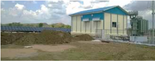
Fig. 17: Solar Inverter room by Smart Built Prefab Private Limited, Nellore [16]
