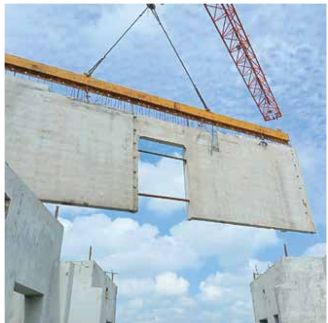
Fig.12: Placement of Walls
