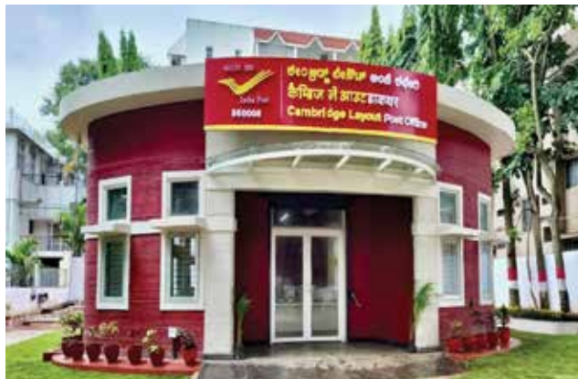
Fig. 14 b): Post Office Building, Bangalore [13]
