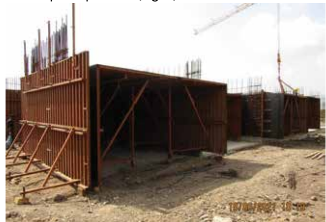
Fig. 4: Installation of Tunnel Formwork
