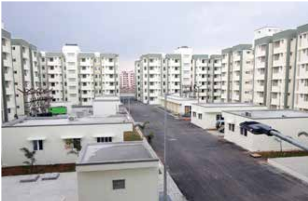
Fig.3: Completed Light House Project at Chennai
