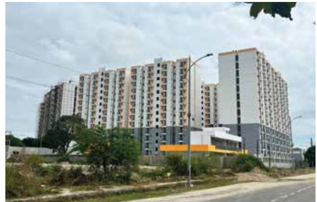
Fig.10: Completed buildings of Light House Project at Lucknow
