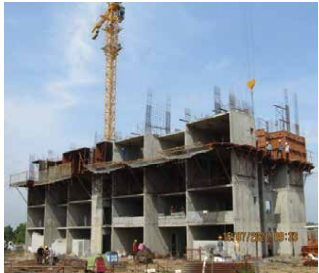
Fig.5: Tunnelform placing and casting of concrete
