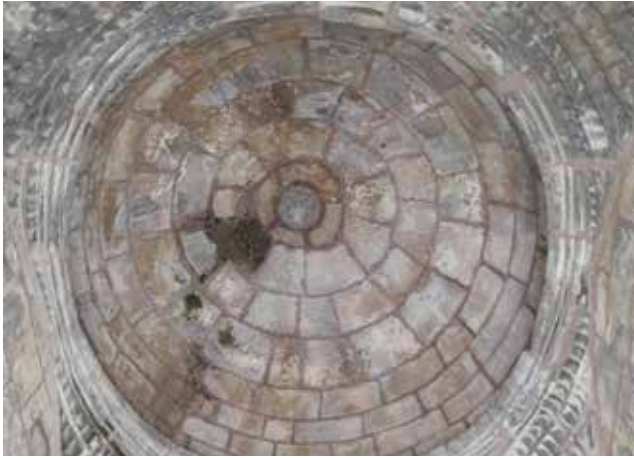
Fig.10: Garh Panchakot Kolkata Temple, Arch inside
