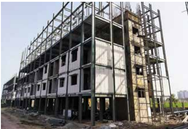
Fig. 7: Placement of Prefabricated Sandwich Panels in Steel Structure Frame
