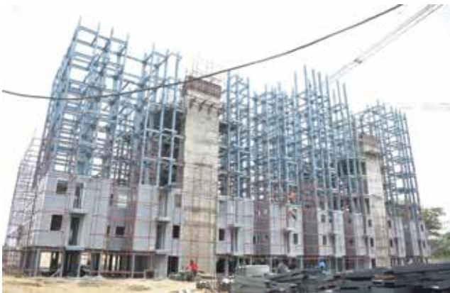
Fig. 9: Placement of PVC Wall Form Panels in Steel Structure Frame
