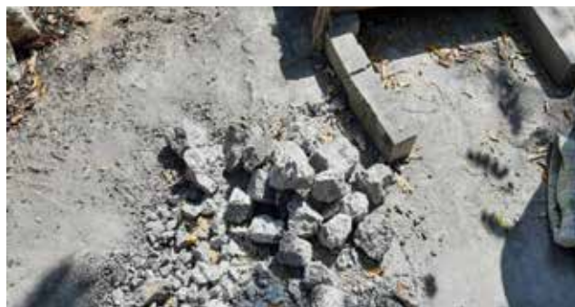
Fig. 2: Collected Recycled Concrete Aggregate (rigid pavement)
