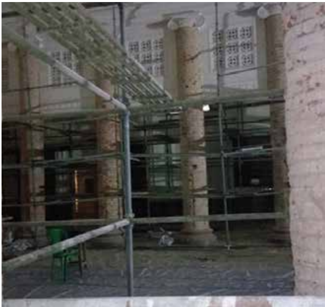
Fig. 5: Restoration work of Town Hall, Kolkata
