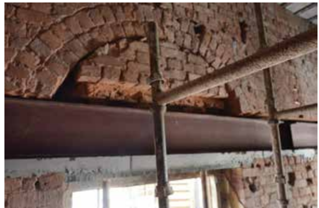
Fig.3: Retrofitting works at Writers Building, Kolkata
