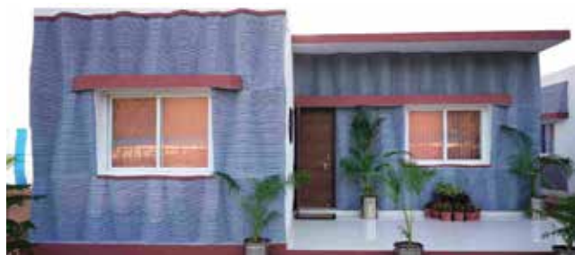
Fig. 13: Housing unit Indian Defence, Indian Air Force - Chiloda, Gujarat. [12]
