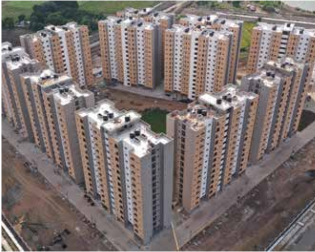
Fig.6: Completed Light House Project at Rajkot
