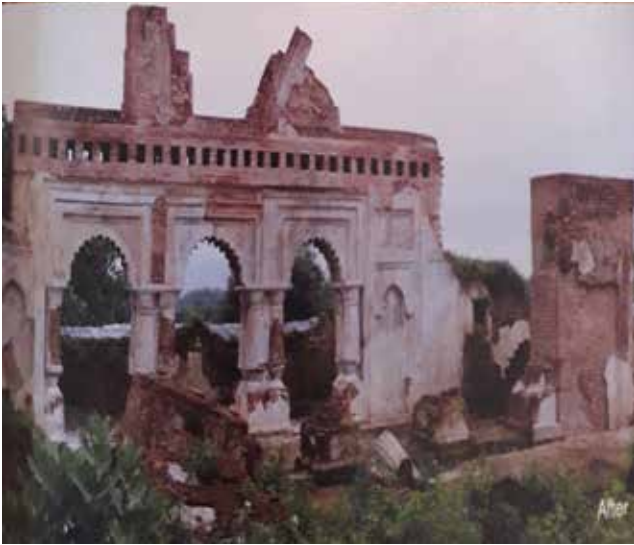
Fig. 11: Restoration of Gate at Rani Mahal Garh Panchakot
