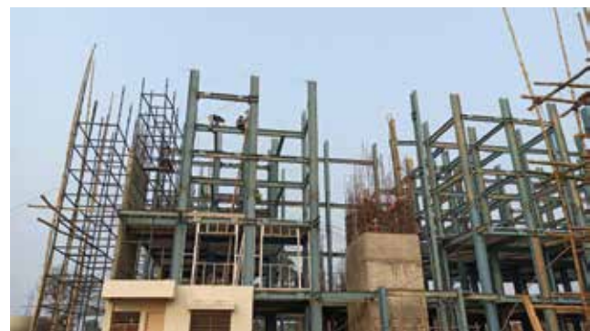
Fig.13: Placement of LGS frames in Steel Structure System
