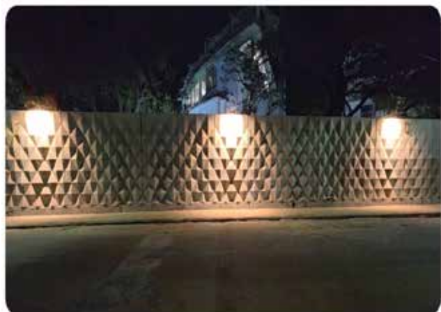
Fig. 11: 3D Printed Wall, Chepauk Cricket Stadium, Chennai [12]
