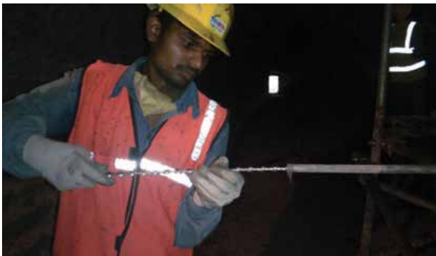
Fig.6: Restoration & Retrofitting works in Town Hall
