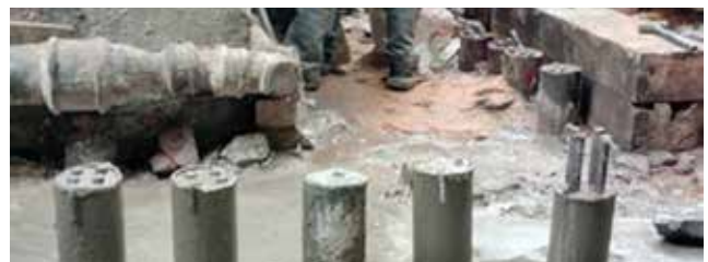
Fig. 8: Micro piling works for stabilisation of soil movement
