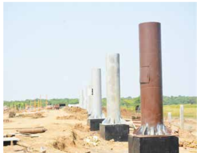
Fig. 5. Erection of Trunk
