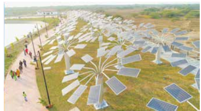
Fig. 8. A view of complete Solar Trees
