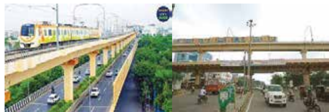
Longest Double-Decker Flyover
