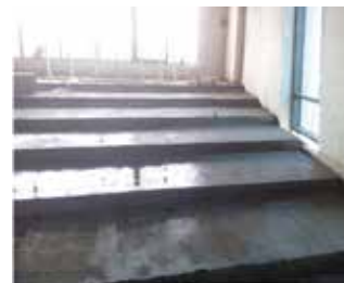
EPS Geofoam blocks laid in lecture hall of NISM
