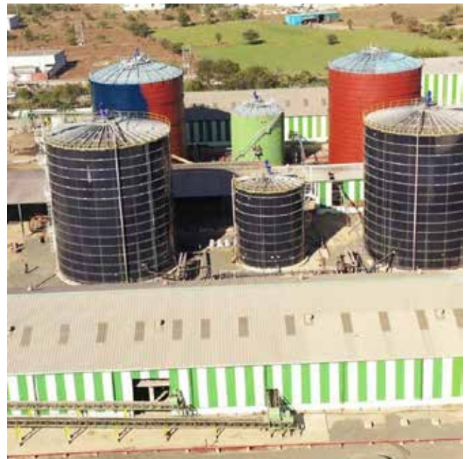
Bio CNG Plant at Indore
