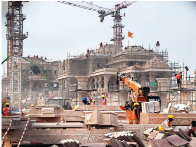
Ram Temple under construction
