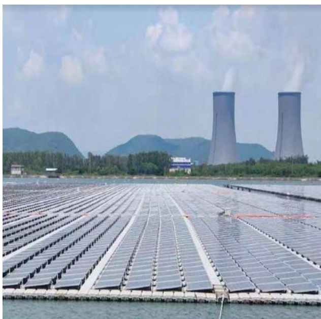
Fig.: India's Largest Floating Solar Power Plant of 25MW capacity
