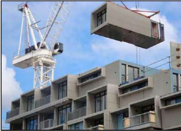
Fig. 2 Prefabricated Prefinished Volumetric Construction
