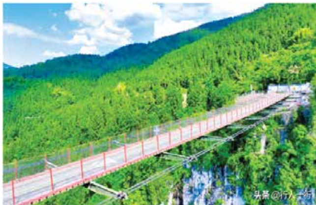
Dadong River Bridge
