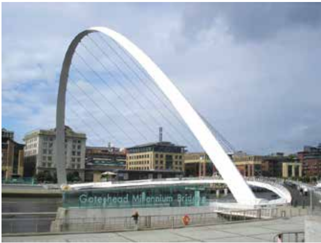
Gateshead Millennium Bridge
