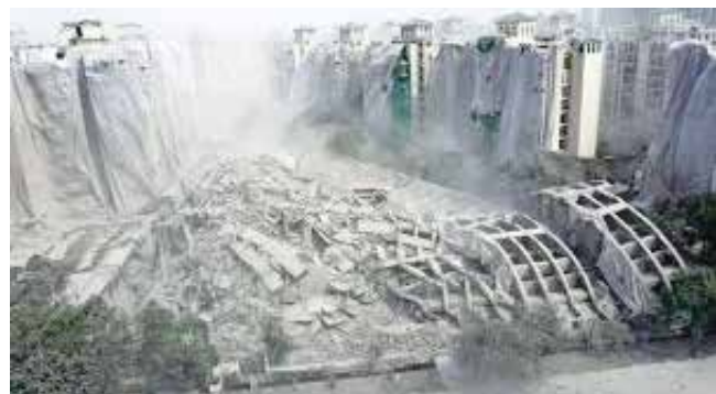
Twin Tower after demolition
