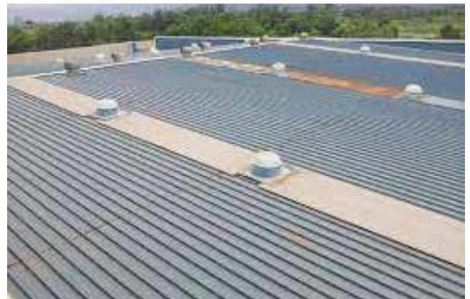
View of Skylights from Top of Roof
