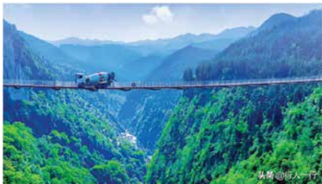
Dadong River Bridge Carrying Heavy Vehicle
