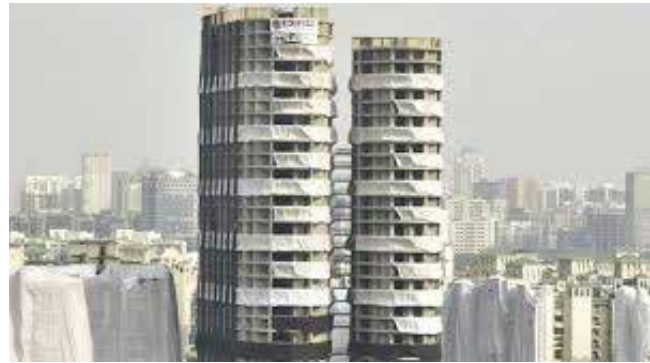
Twin Towers before demolition
