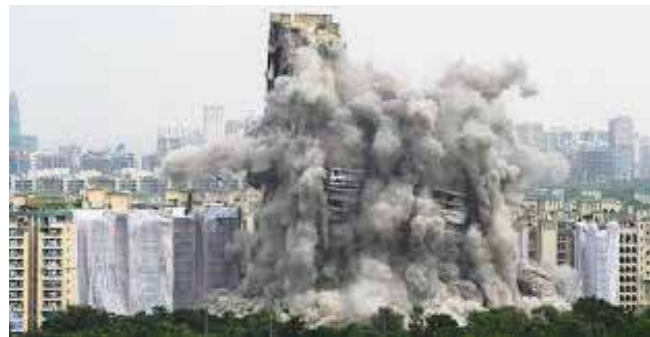
Twin Tower being razed through implosion
