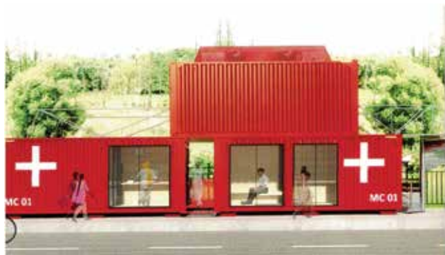
Fig. 7: A primary healthcare centre built out of used shipping containers for Delhi Government Mohalla Clinics programme, Architect Akshat Bhatt
