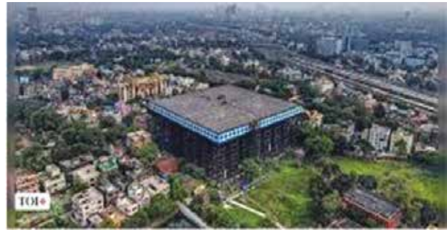
Tala Water Tank, Kolkata
