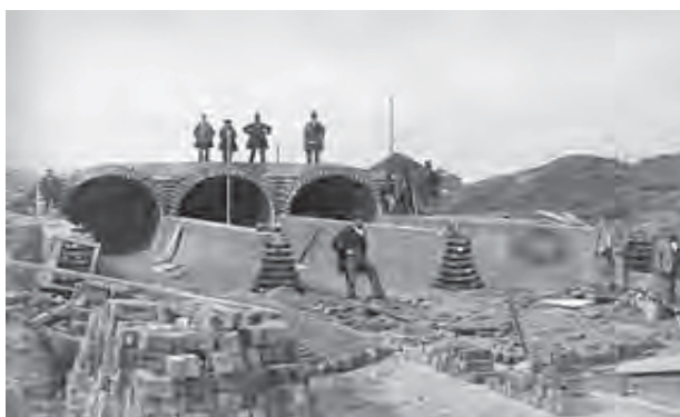
Fig.1 London Sewage System being built in 1860
