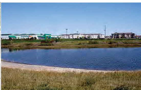
Fig.3 Trounce Pond in Saskatoon, Canada serves as a storm water detention basin within the local drainage system
