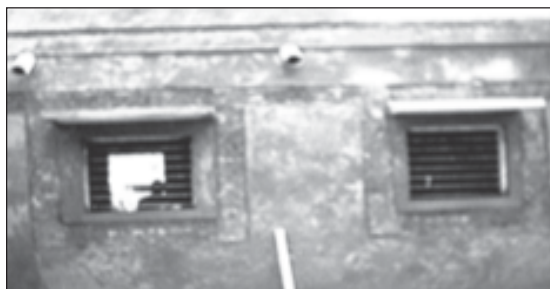
Fig. 6 Seismic Belt around Window Openings
