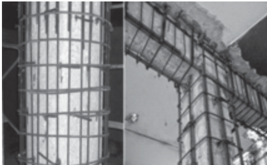
Fig. 1 RCC Jacketing with Shear Keys
