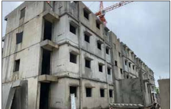
Fig. 6: 3 D Modular Construction at Ranchi
