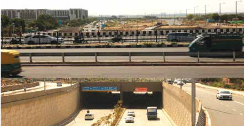
Fig.4: View of the underpass below NH-8
