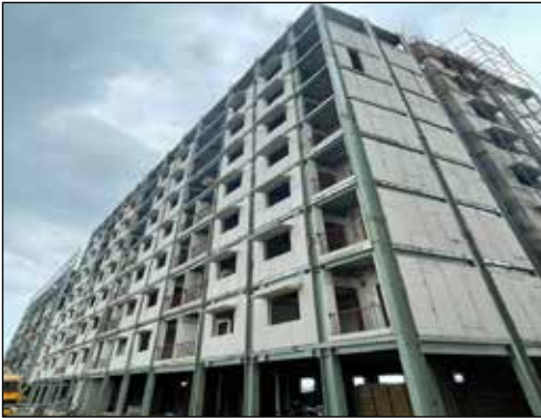
Fig. 3: Sandwich Panel System Construction at Indore
