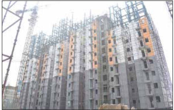
Fig. 4: Stay in place Formwork Construction at Lucknow
