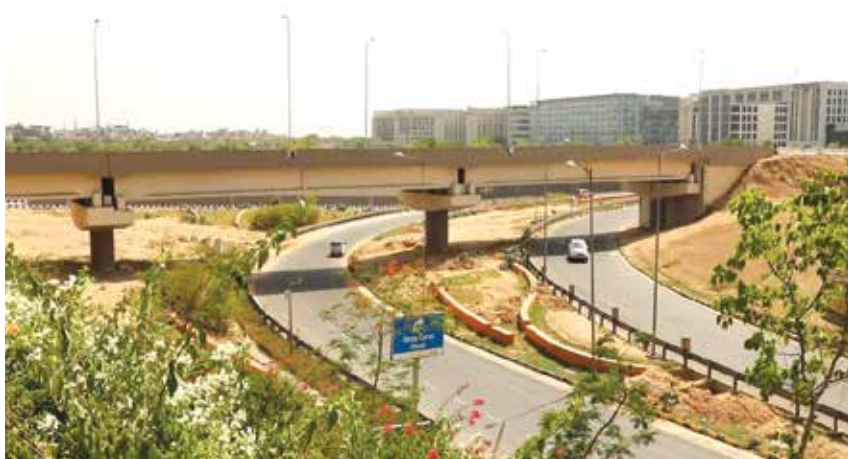
Fig.8: Bridge in front of existing tunnels of Airport
