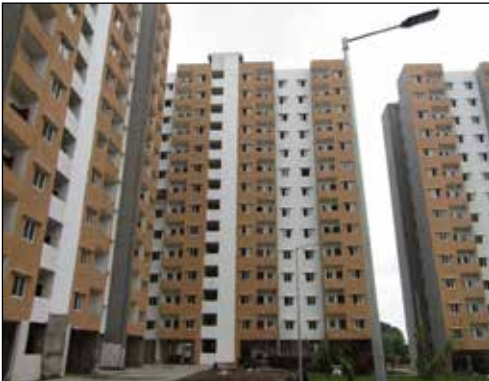
Fig. 5: Monolithic Concrete Construction at Rajkot
