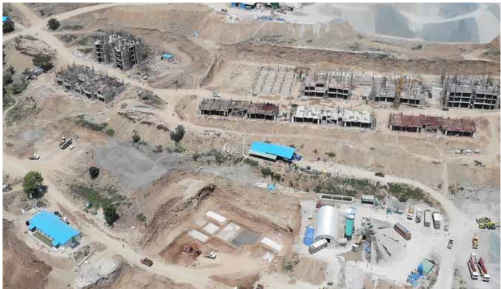
Fig. 3: An Aerial View of the Works in Progress at Awantipora
