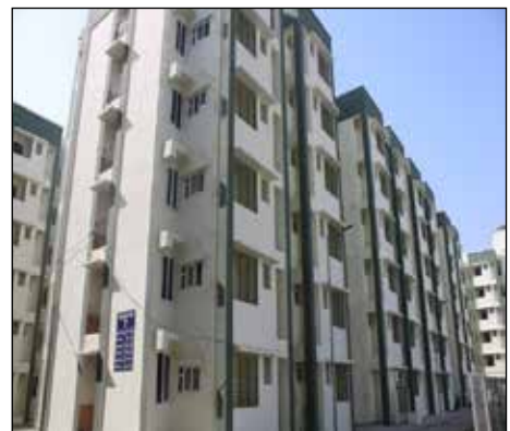
Fig. 2: Pre-cast Concrete Construction at Chennai
