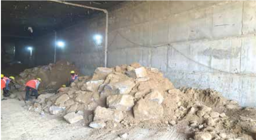
Fig.2: Rocks being excavated and brought out of Underpass
