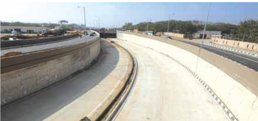
Fig.6: View of the ramps of the underpass
