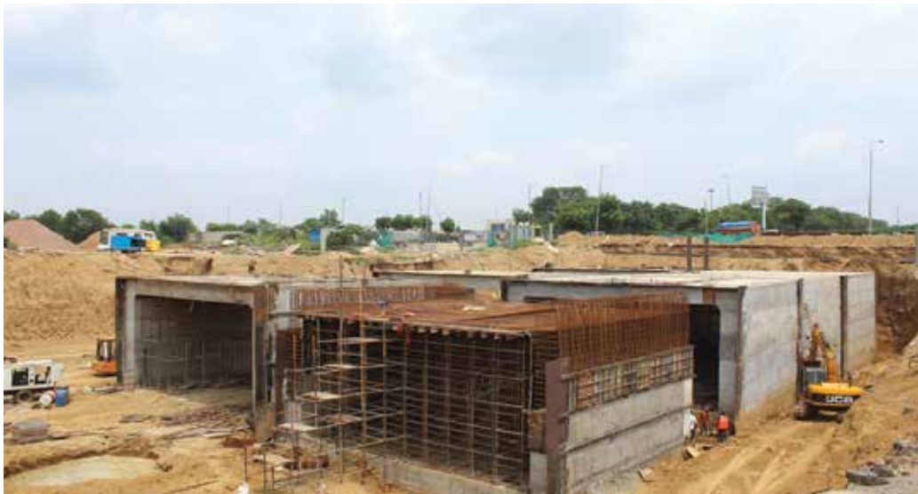
Fig.1: Construction of Boxes for Underpass
