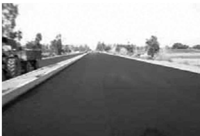
**Fig. 5: Finished Surface of Plastic Waste Modified Mix at Rohtak-Bhiwani Road**
