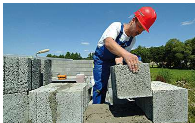
Fig. 10: LWA Blocks for Masonry
