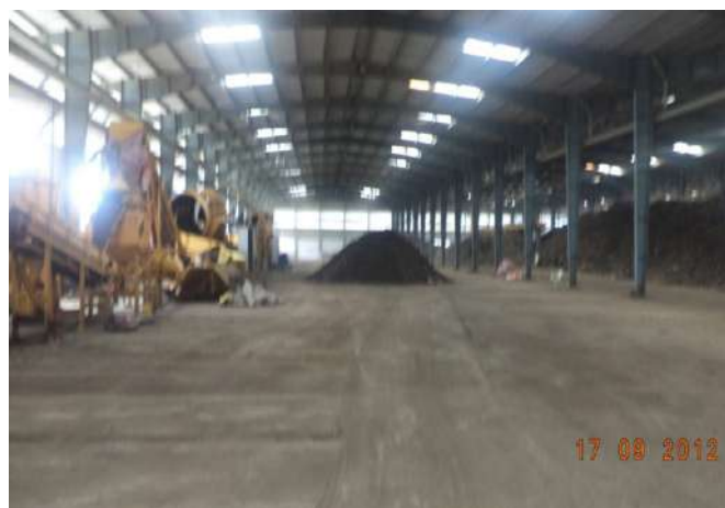
Fig. Composting Facility at Bawana
