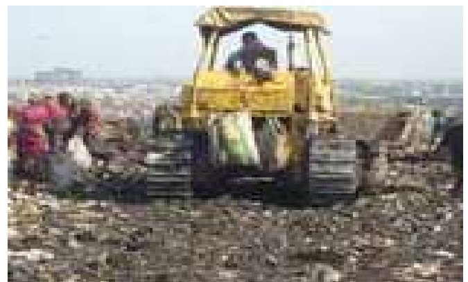
Fig. Sanitary Land Fill Site at Bhalswa
