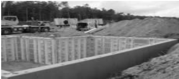
Fig. 4: Precast Concrete Foundations
