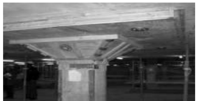
Fig.3: Flat Slab Construction
