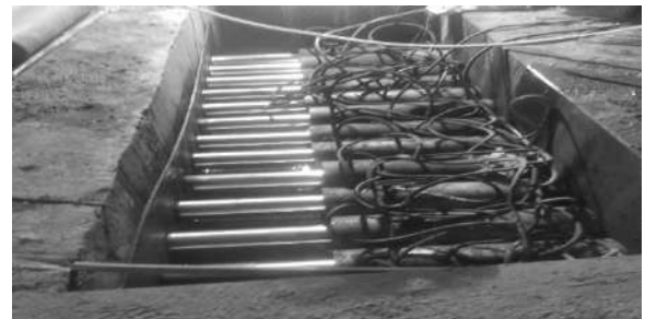
Fig.10: Pushing of Box Segments
