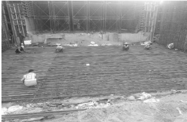
Fig.9: Reinforcement for Box Section
