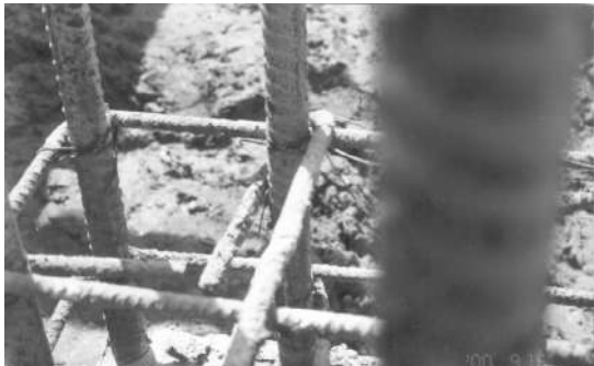
Fig.15: Seismic Detailing of Transverse Reinforcement
