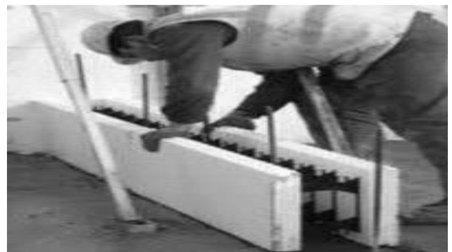
Fig.7: Insulating Concrete Formwork
