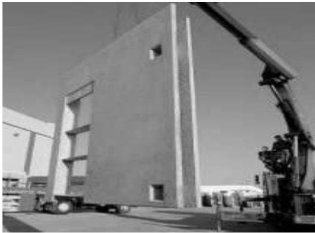
Fig.1: Precast Flat Panel System
