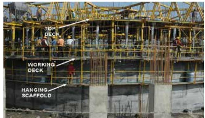
**Fig. 26: Slip Forming in Progress**
