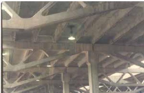
**Fig. 11: Close Up View of Precast Trusses
