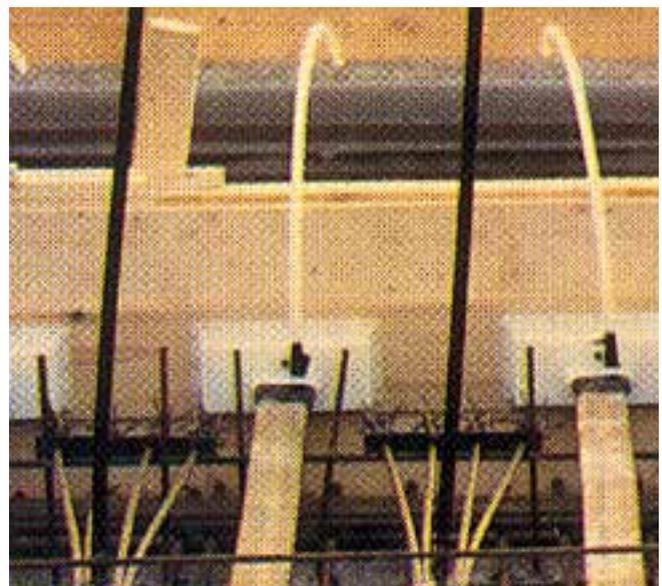
**Fig. 9: Flat Pre-stressing Cables**
