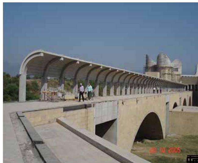
**Fig.3: Precast Concrete Canopy Over Pedestrian Bridge**
