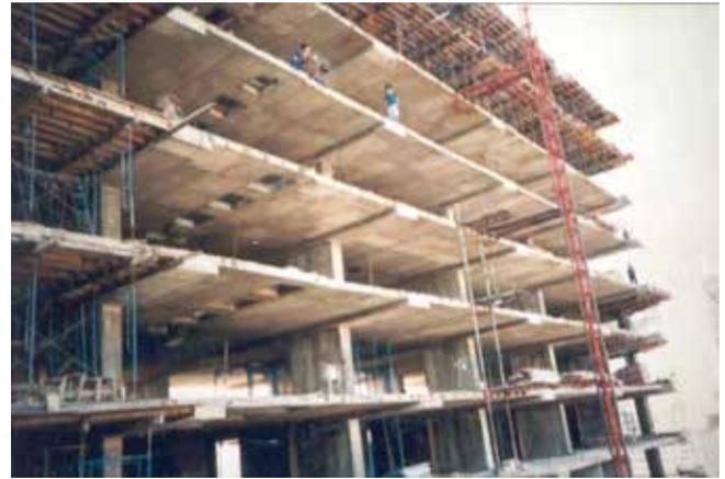
**Fig. 8: Pre-stressed Banded Slabs**
