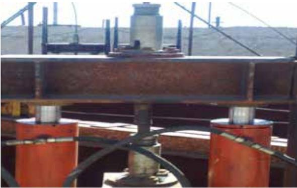
**Fig. 29: Strand Jacks for Lifting Flues**
