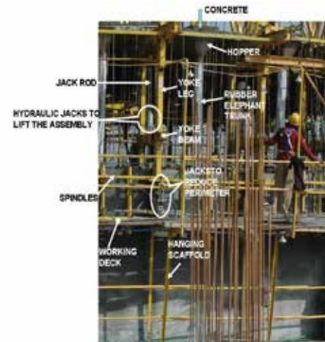
**Fig. 27: Slip Forming Equipment**
