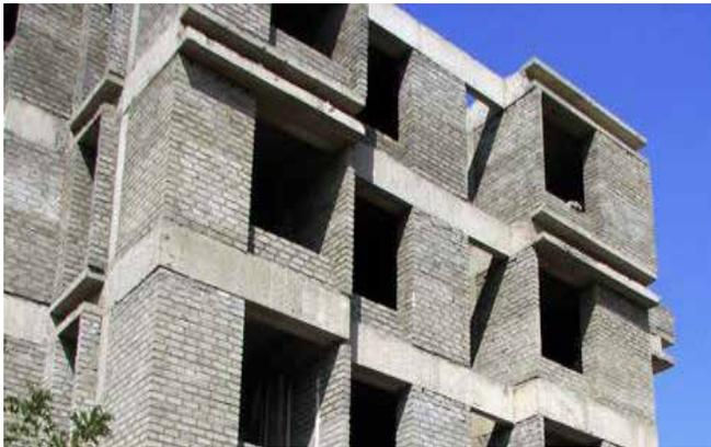
**Fig. 4: Building Made of Fly Ash Bricks**
