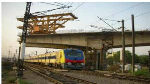
**Fig. 14 : Cantilever Construction Over Railways**
