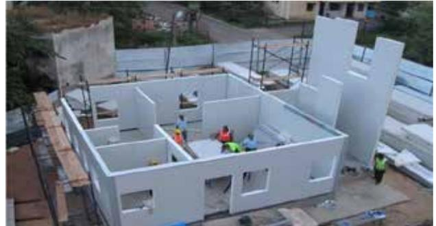
**Fig.1: Installation of SIP**
