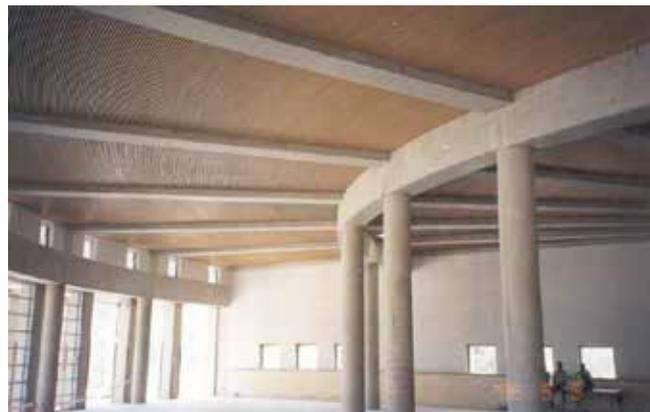
**Fig. 2: Fair Faced Concrete Beams Visible Below False Ceiling**
