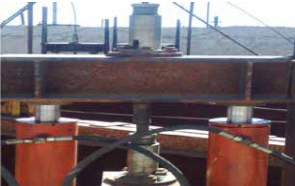
**Fig. 29: Strand Jacks for Lifting Flues**
