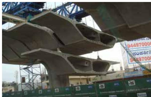
**Fig. 18 : Segments Suspended from Launching Girder**
