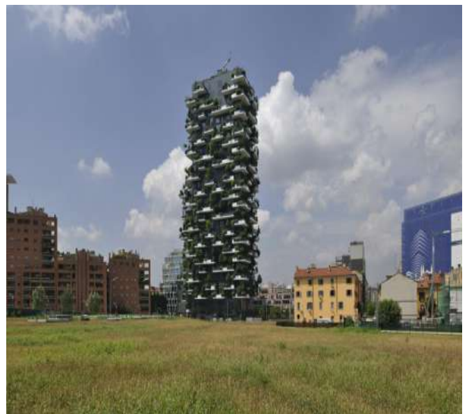
Fig. 4: Bosco Verticale Building
