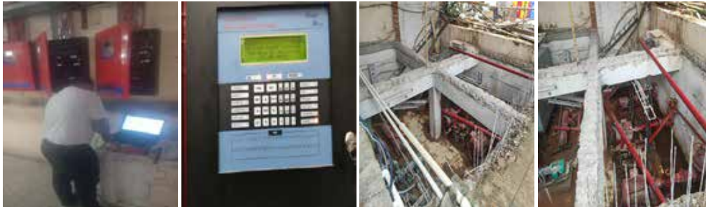
Fig. 3: The fire control module being installed Successfully after programming to properly Number and loop the detection system
