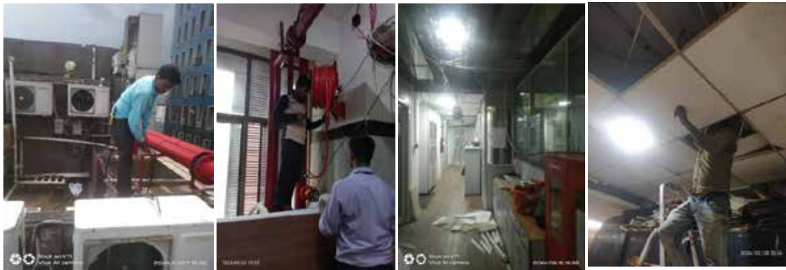
Fig. 1: Installation of Fire hydrant lines, branch/sprinkler lines and hose reel pipe
