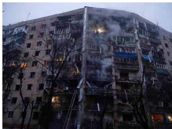
Fig. 1: Damaged Apartment Building in Residential Neighborhood at Kramatorsk, Donetsk Region (Ukraine) dated Feb. 8, 2026.
