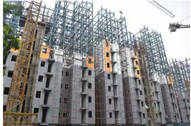
Fig. 2: Stay in Place Panels for infill Walls
