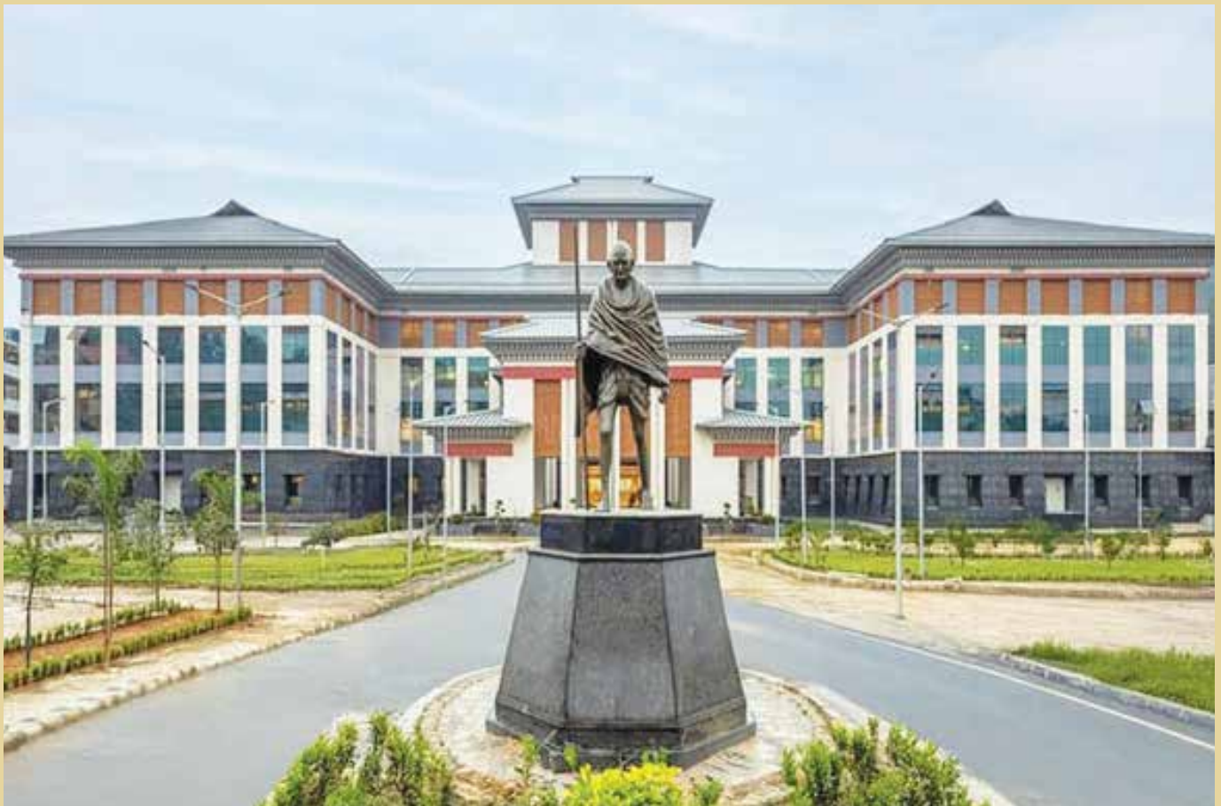
Gauhati High Court's Itanagar Permanent Bench Building at Naharlagun, Arunachal Pradesh
