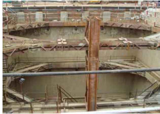
Challenge: unbalanced earth pressure TBM launching shaft
