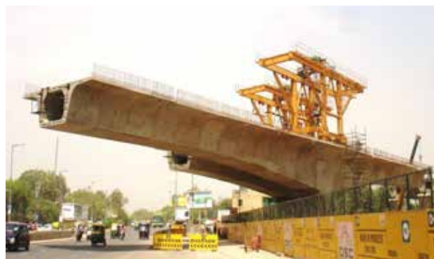
Barapulla Long Spans: Simultaneous Progress of both carriage ways by cantilevering
