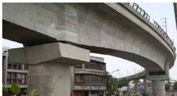
Cast-In-Situ 4-Span Segmental Construction (38.5M+55.0M+38.5M+38.5M)
