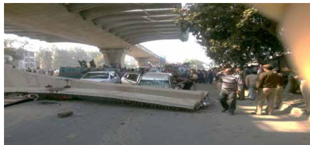
Collapse of Wing in Construction Stage
