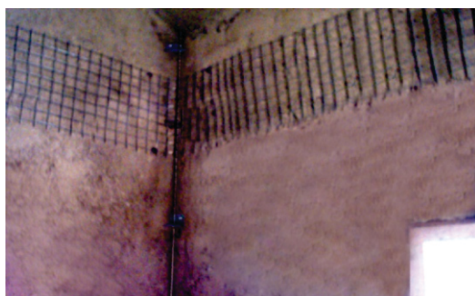
Fig. 6 Vertical Reinforcement at Interior Corner
