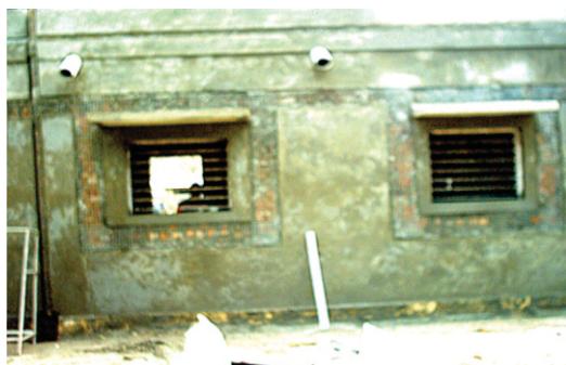
Fig. 4 Seismic Belt around Window Openings
