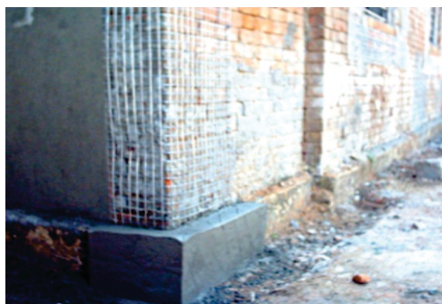
Fig.5 Seismic Belt at External Corner
