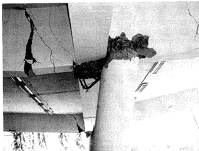
Figure 40 Failures in beam and column (Andaman earthquake, 2004)
