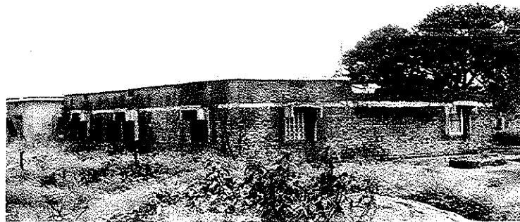
Figure 16 Good integral action in a masonry building with lintel band (after Latur earthquake, 1993) (Source: www.nicee.org )
