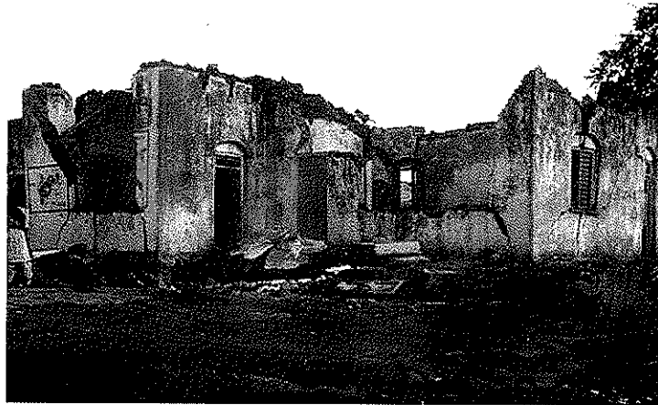
Figure 15 Poor integrity in a masonry building (after Latur earthquake, 1993) (Source: www.nicee.org )
