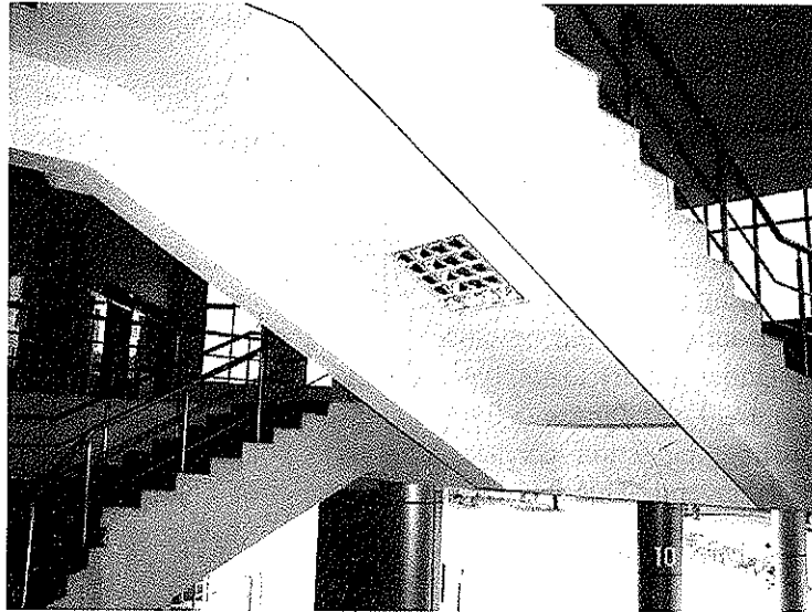
Figure 42 Stairs with stringer beams connected to the building frame
