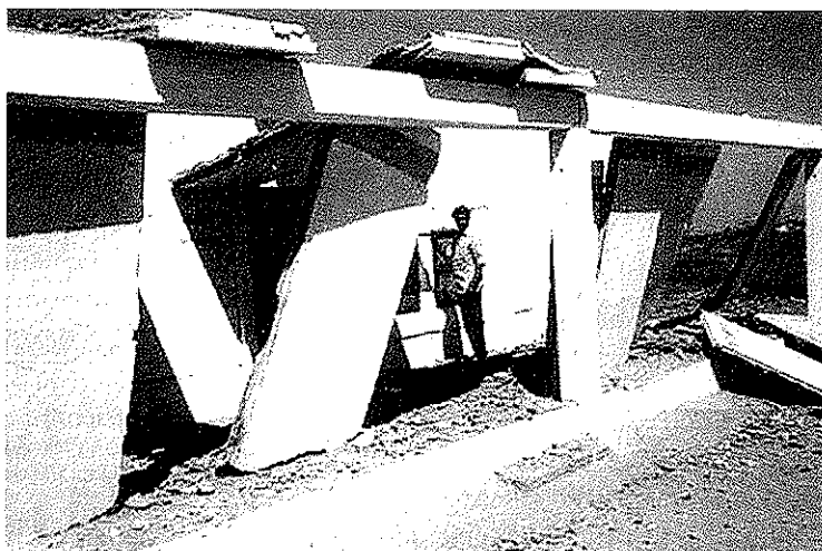
Figure 43 Lack of proper connection in a pre-cast building (after Bhuj earthquake, 2001) (Source: www.nicee.org )
