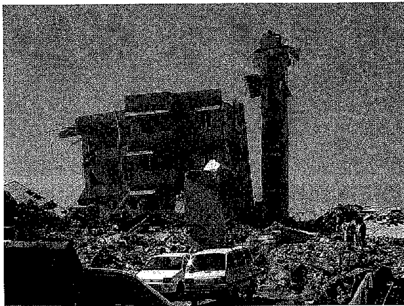
Figure 17 Lack of integrity between lift core and rest of the building (after Bhuj earthquake, 2001) (Source: www.nicee.org )
