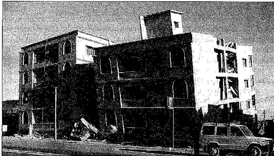
Figure 10 Collapse of the ground storey of a building (after Bhuj earthquake, 2001) (Source: www.nicee.org )
