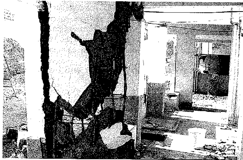
Figure 39 A shear failure in a column (after Bhuj earthquake, 2001) (Source: www.nicee.org )
