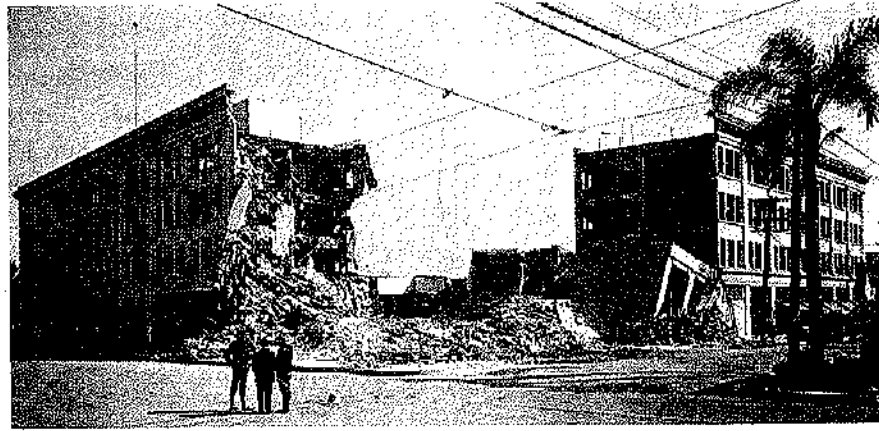
Figure 19 Collapse of an "L" shaped building (after Skopje earthquake, Macedonia, 1963)
