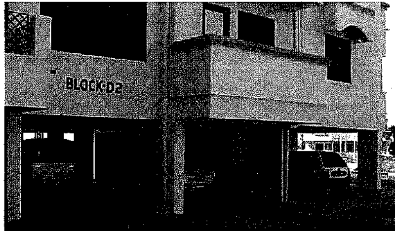
Figure 22 Building with open ground storey (Source: www.nicee.org )
