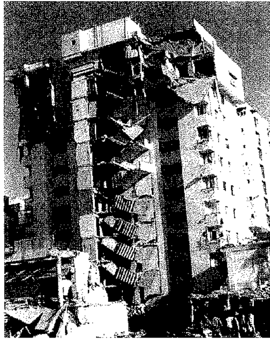
Figure 27 Collapse of stair slabs (after Bhuj earthquake, 2001) (Source: www.nicee.org )
